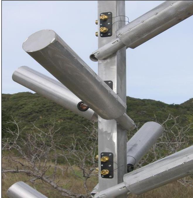
**Figure 4.3** Close-up of spark arrestors
